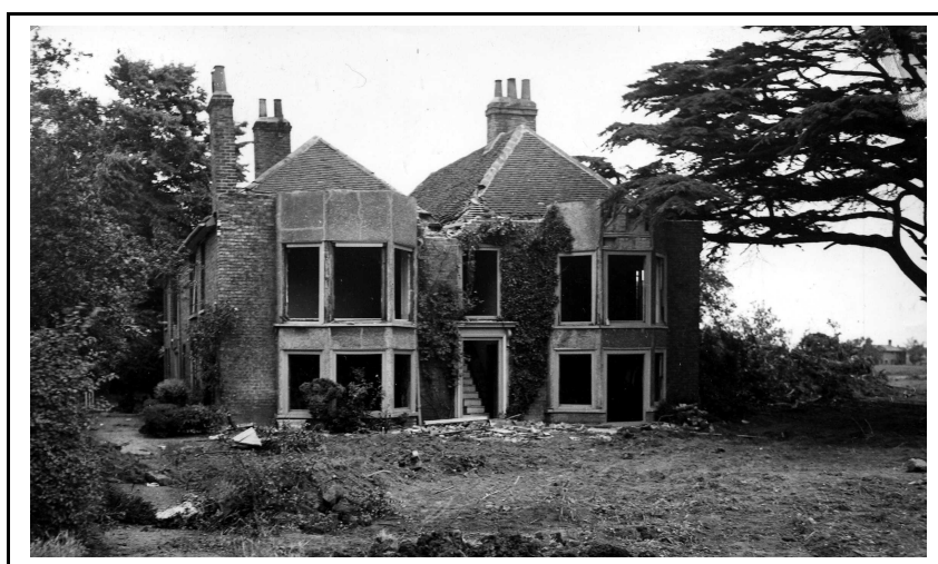
Demolition of Heathrow Hall 1944
